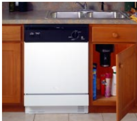
OFFSET INSTALLATION FOR USE WITH DISPOSER
