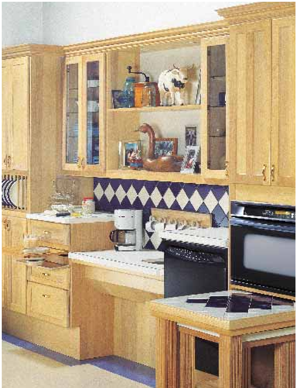
Wall ovens, cooktops, microwaves and dishwashers can be installed at varying heights to maximize accessibility.
