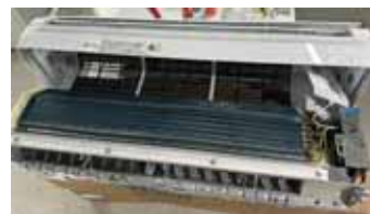
3. Remove the cover by removing these 10 screws.
