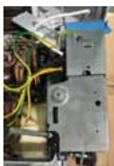
4. Remove the electrical box cover.
