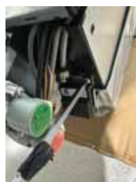
5. Remove leak sensor.
