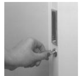
Built-in lock with self-ejecting key
